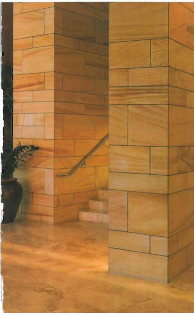
In addition to the Indian sandstone, the interior spaces utilize travertine flooring.
